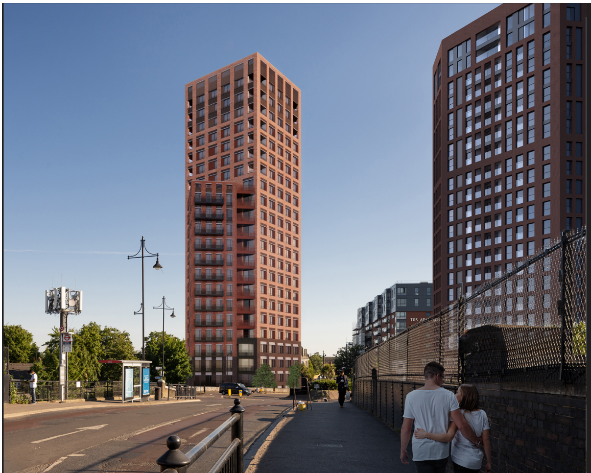
View of Proposed Building from North with approved Kings House Scheme indicated on right
